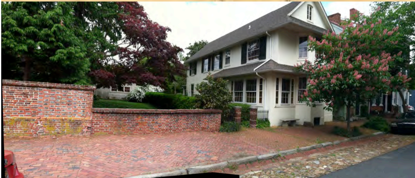
Arch, water table, glazed header flemish bond
